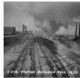
CPR Station and Coach Yard - Showing Heating ...
