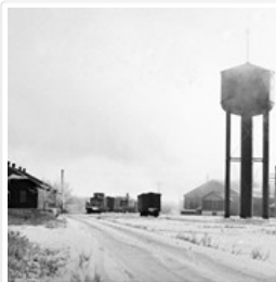
CPR Shop Buildings, Water Tower, and Bunkhouse
