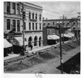
Sewer pipe installation along 700 block of Rosser ...
