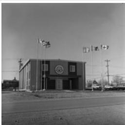
Dakota-Ojibway Tribal Council Building
