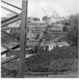
Demolition of Second First Street Bridge
