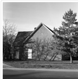
Masonic Temple (appears to be a former church), ...
