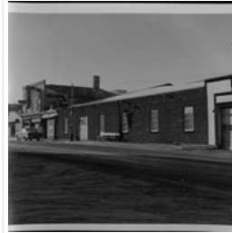
West side 200-block 10th Street facing south from ...
