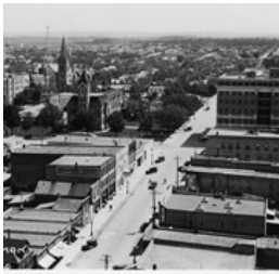
9th Street aerial view facing south, Brandon, Manitoba
