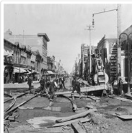
Brandon Municipal Railway Construction
