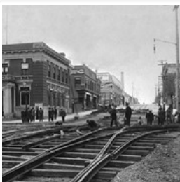
Brandon Municipal Railway Construction
