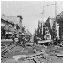
Brandon Municipal Railway Construction
