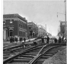
Brandon Municipal Railway Construction
