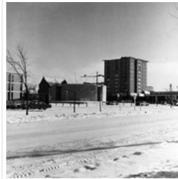
Brandon University - McMaster Hall Construction
