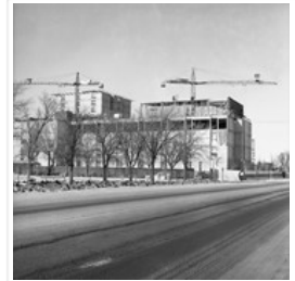
Brandon University - Brodie Science Centre Construction
