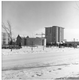
Brandon University - McMaster Hall construction
