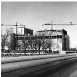
Brandon University - Brodie Science Centre Construction
