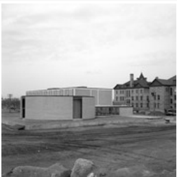
Brandon College - old and new buildings
