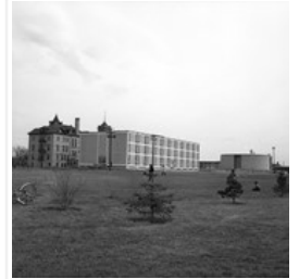
Brandon College - old and new buildings
