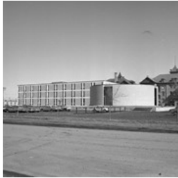
Brandon College - old and new buildings
