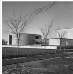
Brandon College - old and new buildings
