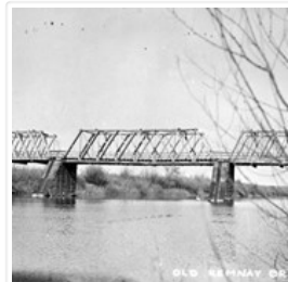
Assiniboine River Bridge North of Kemnay
