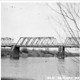
Assiniboine River Bridge North of Kemnay
