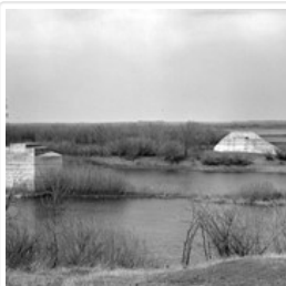
Grand Trunk Pacific Bridge Piers
