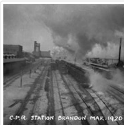
CPR Station and Coach Yard - Showing Heating ...
