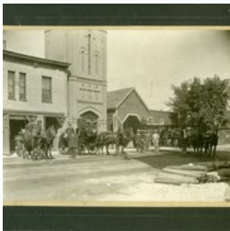
Original Fire Hall
