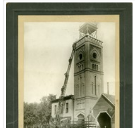
Original Fire Hall
