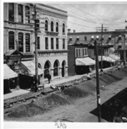
Sewer pipe installation along 700 block of Rosser
