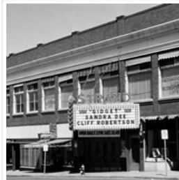
Hughes Block (Strand Theatre building)
