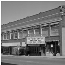
Hughes Block (Strand Theatre building)
