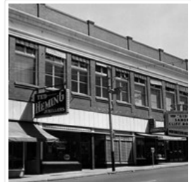
Hughes Block (Strand Theatre building)
