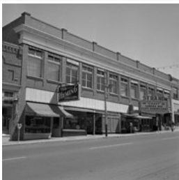
Hughes Block (Strand Theatre building)
