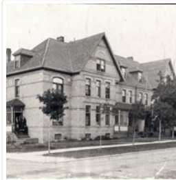
Hughes residential property - Lorne Terrace
