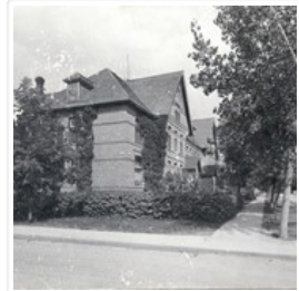
Hughes residential property - Lorne Terrace
