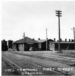
CNR Engine Terminal
