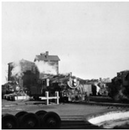
CNR Engine Terminal
