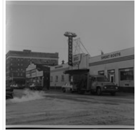
Greyhound Bus Depot, 11th Street and Princess Avenue, ...
