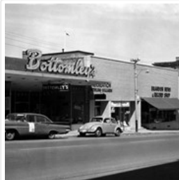
10th Street Businesses - West Side of 100 ...
