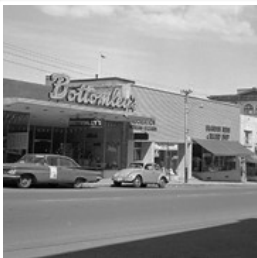
10th Street Businesses - West Side of 100 ...
