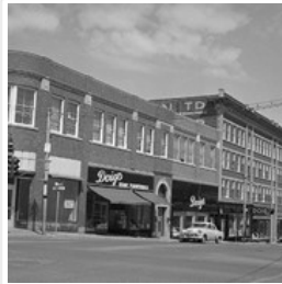
10th Street Businesses - West Side of 100 ...
