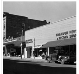
10th Street Businesses - West Side of 100 ...
