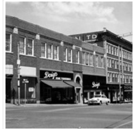
10th Street Businesses - West Side of 100 ...
