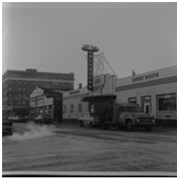
Greyhound Bus Depot, 11th Street and Princess Avenue, ...
