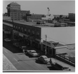
East side 10th Street facing north from Princess ...
