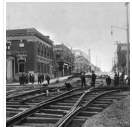
Brandon Municipal Railway Construction
