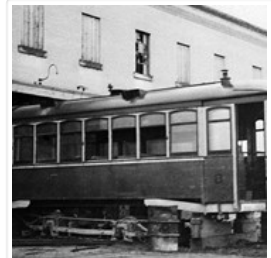
Dismantling of Streetcar No. 8
