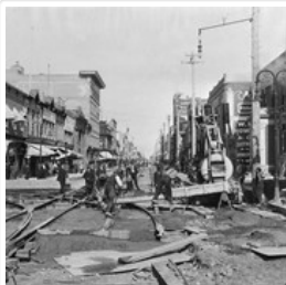
Brandon Municipal Railway Construction
