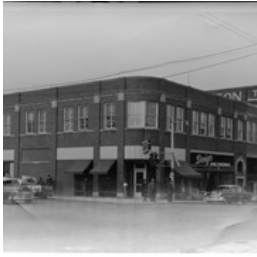
Hughes Building, Brandon, Manitoba
