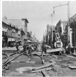
Brandon Municipal Railway Construction
