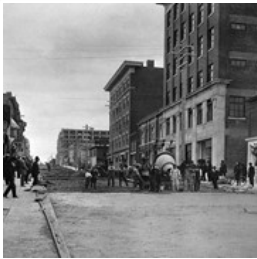
Paving Ninth Street
