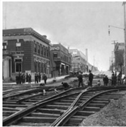
Brandon Municipal Railway Construction
