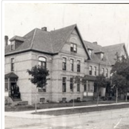
Hughes residential property - Lorne Terrace
