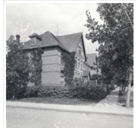
Hughes residential property - Lorne Terrace
