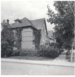
Hughes residential property - Lorne Terrace
