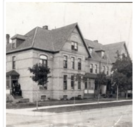
Hughes residential property - Lorne Terrace
