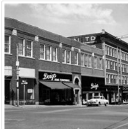
10th Street Businesses - West Side of 100 ...
