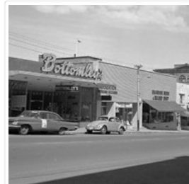
10th Street Businesses - West Side of 100 ...
