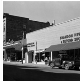
10th Street Businesses - West Side of 100 ...
