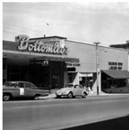
10th Street Businesses - West Side of 100 ...
