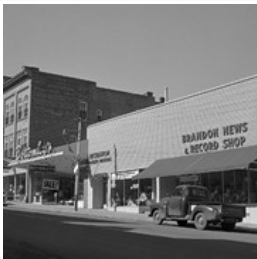
10th Street Businesses - West Side of 100 ...
