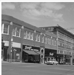
10th Street Businesses - West Side of 100 ...
