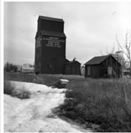
Grain elevators, Hartney, Manitoba
