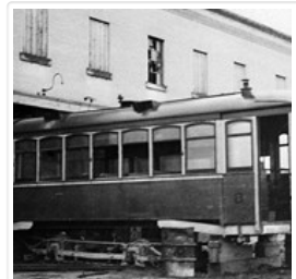
Dismantling of Streetcar No. 8
