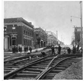
Brandon Municipal Railway Construction
