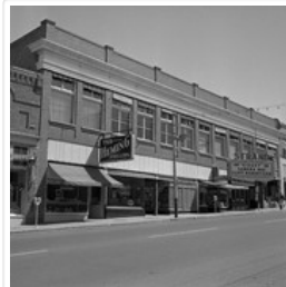
Hughes Block (Strand Theatre building)
