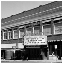
Hughes Block (Strand Theatre building)
