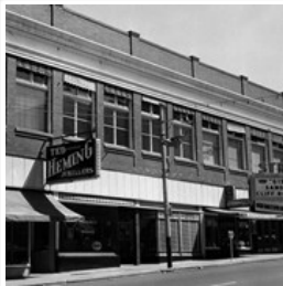
Hughes Block (Strand Theatre building)
