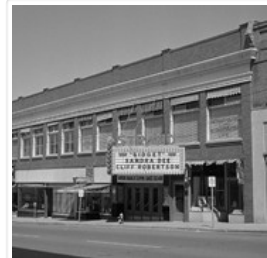
Hughes Block (Strand Theatre building)
