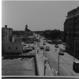
Princess Avenue facing east from 10th Street, Brandon, ...
