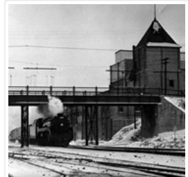
CPR "Dominion" Under First Street Bridge
