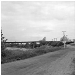
Construction of third First Street bridge
