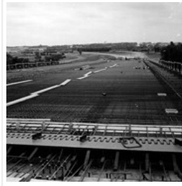
Construction of third First Street bridge
