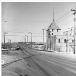
Second First Street bridge
