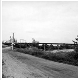
Construction of third First Street bridge
