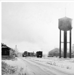
CPR Shop Buildings, Water Tower, and Bunkhouse
