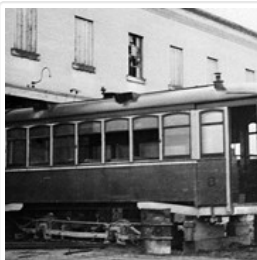
Dismantling of Streetcar No. 8
