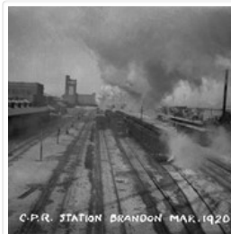
CPR Station and Coach Yard - Showing Heating ...
