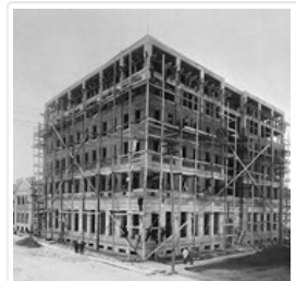
Prince Edward Hotel Construction
