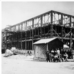
Construction of Parkview Apartments
