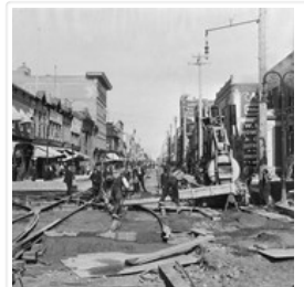
Brandon Municipal Railway Construction
