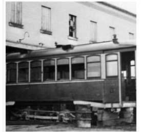
Dismantling of Streetcar No. 8
