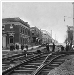
Brandon Municipal Railway Construction
