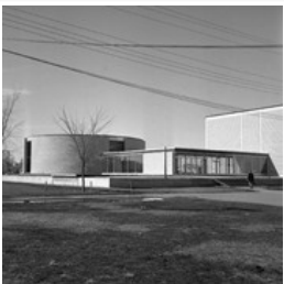
Brandon College - old and new buildings
