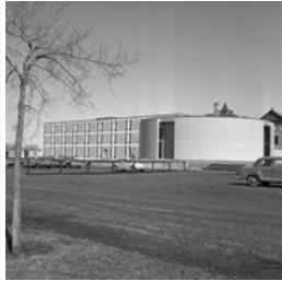
Brandon College - old and new buildings
