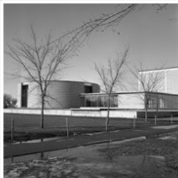
Brandon College - old and new buildings
