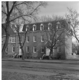
St. Augustine's Roman Catholic Church Offices
