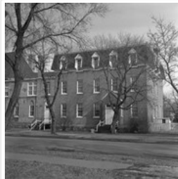
St. Augustine's Roman Catholic Church Offices
