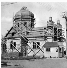
Construction of St. Mary's Ukrainian Catholic Church
