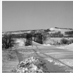
Iron Bridge over Little Saskatchewan River
