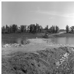
New Culvert and Causeway Across Assiniboine River
