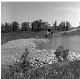
New Culvert and Causeway Across Assiniboine River
