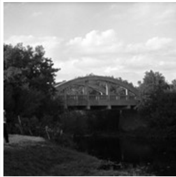
Willow Creek Bridge
