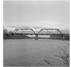
Second 18th Street bridge
