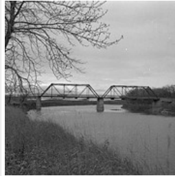
Second 18th Street bridge
