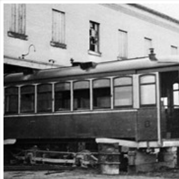
Dismantling of Streetcar No. 8
