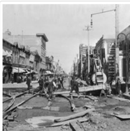
Brandon Municipal Railway Construction
