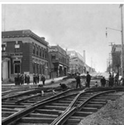
Brandon Municipal Railway Construction
