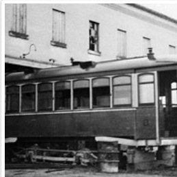
Dismantling of Streetcar No. 8
