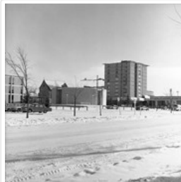
Brandon University - McMaster Hall construction
