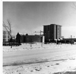
Brandon University - McMaster Hall Construction
