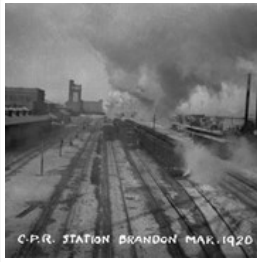
CPR Station and Coach Yard - Showing Heating ...
