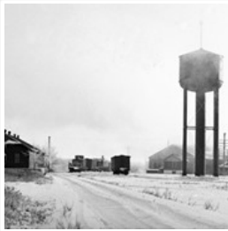
CPR Shop Buildings, Water Tower, and Bunkhouse
