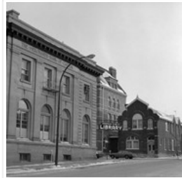
Merchants Bank of Canada Buildings
