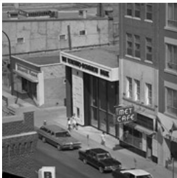
Brandon from roof of Christie Building
