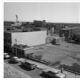
Northeast view from 100 block of Tenth Street
