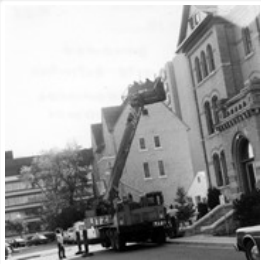
Brandon College Building roof renovations
