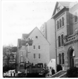
Brandon College Building roof renovations
