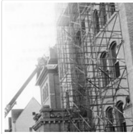
Brandon College Building roof renovations
