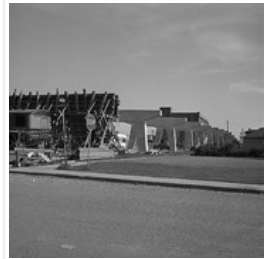
Eighteenth Street Overpass Construction
