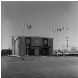
Dakota-Ojibway Tribal Council Building
