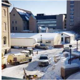
Brandon University campus construction
