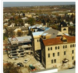
Brandon University campus construction
