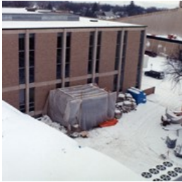
Brandon University campus construction
