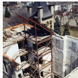
Brandon University campus construction
